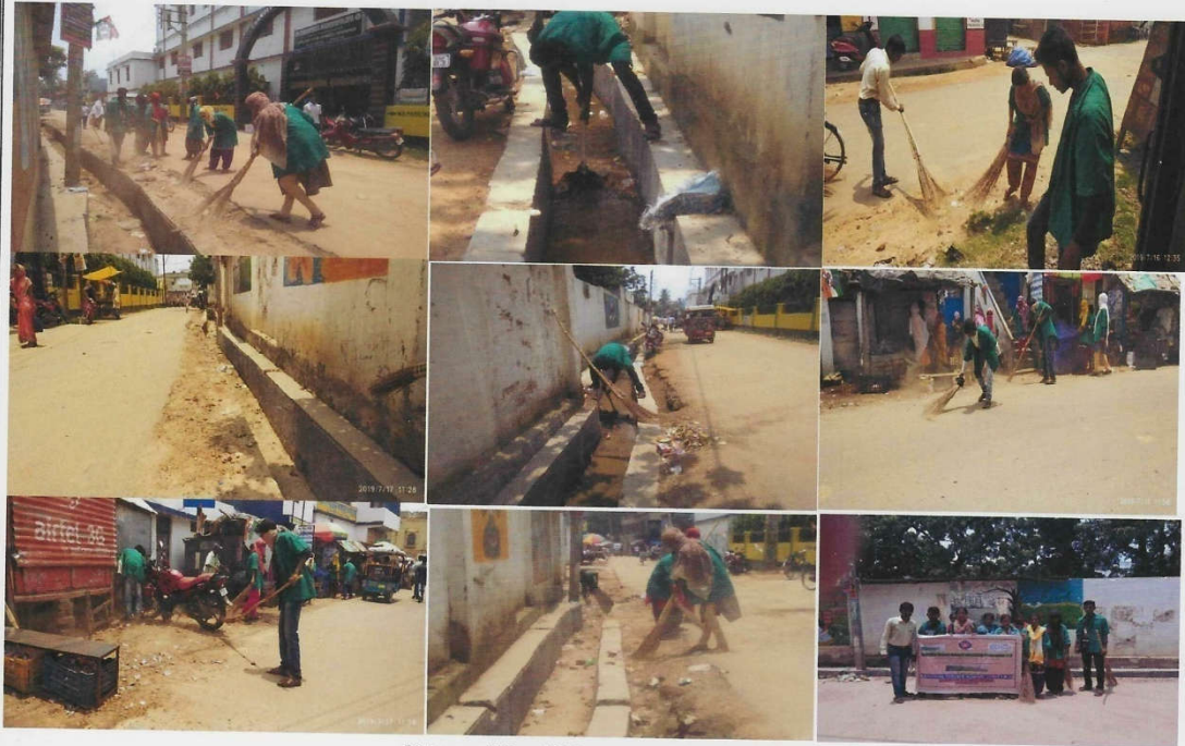
Pictures of Road & Drainages Cleaning 2.0
